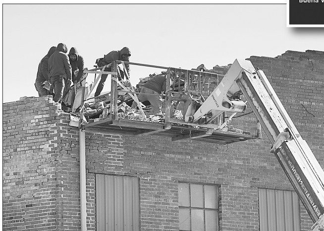
Roofers at work Saturday.
